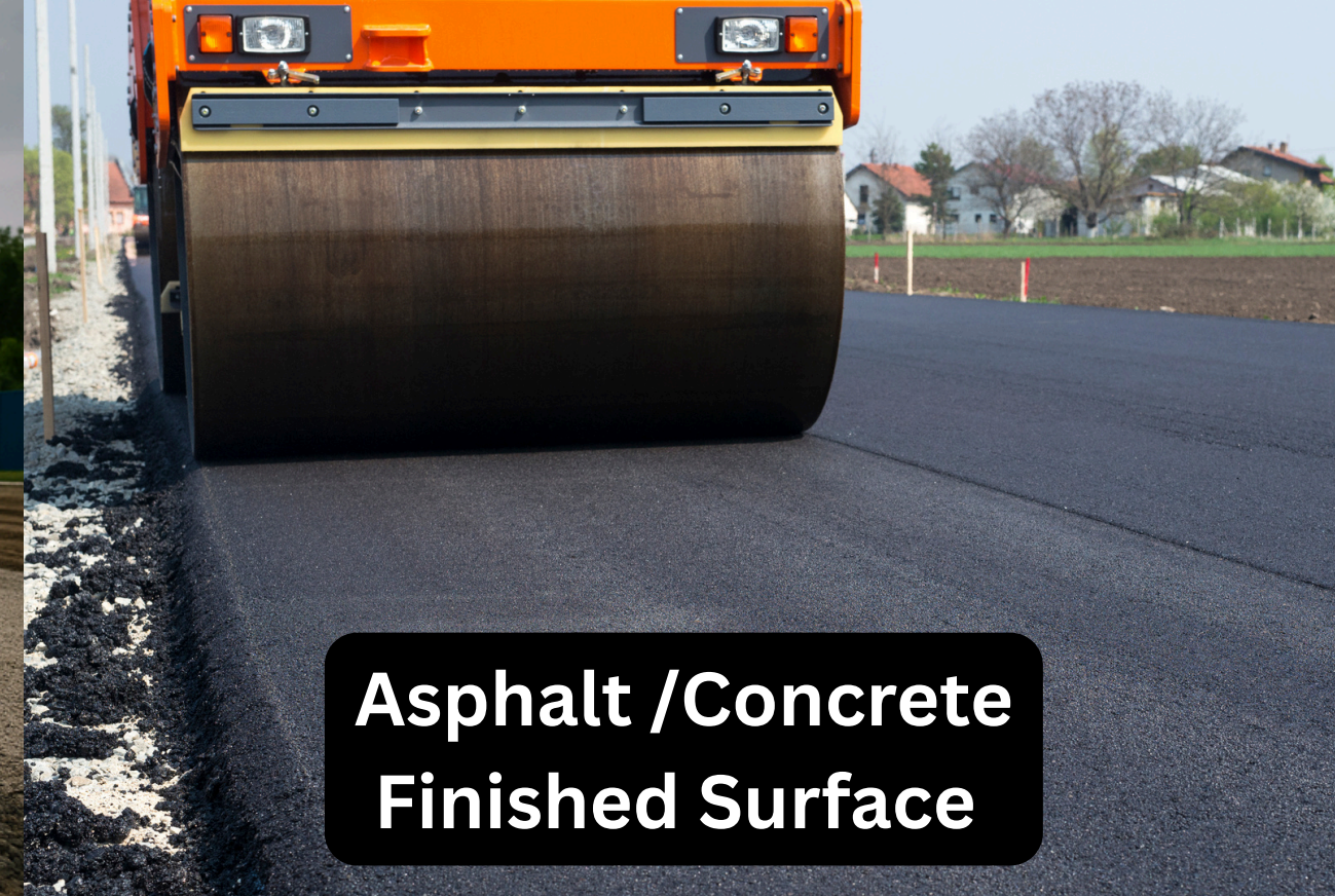
Compaction and Surface Leveling
